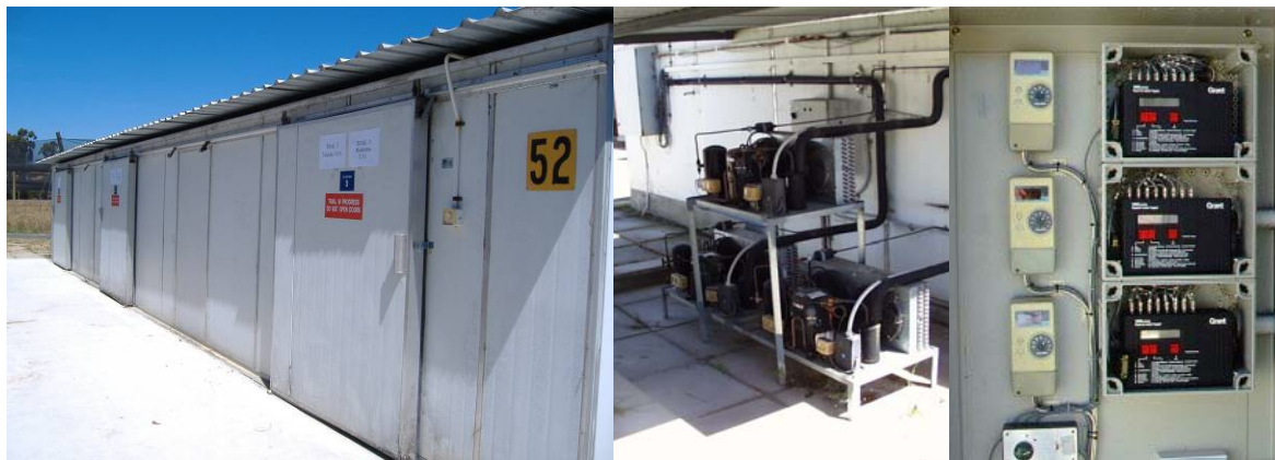
Figure 1 Building 52 houses three cold rooms #3, #4, #5, for 3 replicated cold disinfestation trials to be done simultaneously. View of refrigeration units - there is a separate compressor for each cold room. There is a separate thermostat controller and a separate alarm relay for each cold room. Temperatures are measured and logged using Grant Squirrel data loggers Model 1256 Series, one for each cold room. The loggers are connected to the computer via RS 232 C serial interface.
