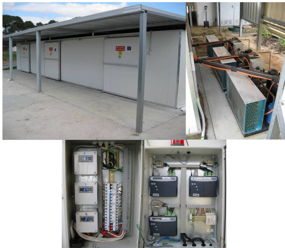
Figure 2 Building 52B houses three cold rooms #6, #7, #8, for 3 replicated cold disinfestation trials to be done simultaneously. View of refrigeration units - there is a separate compressor for each cold room. There is a separate thermostat controller and a separate alarm relay for each cold room. Temperatures are measured and logged using Grant Squirrel data loggers Model 2020 Series, one for each cold room. The loggers are connected to the computer via an Ethernet interface.
