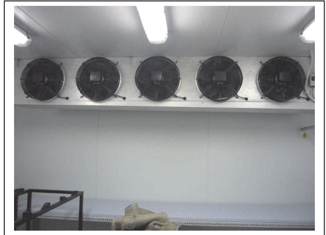
Figure 25 The rear, top cooling fans.
