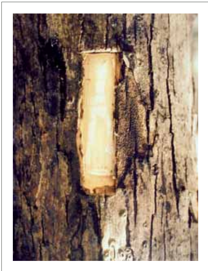
Figure P2. Superficial canker caused by Endothia : the infection has not penetrated the entire thickness of the bark so the cambium remains intact. This type of canker has little impact on stem quality
